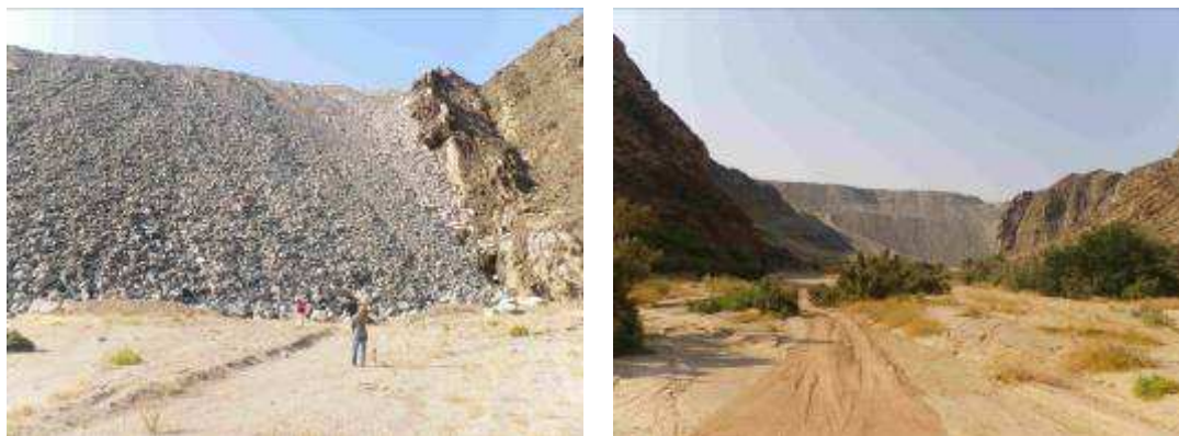
View of the waste rock dump at Dome Gorge (picture taken from the Khan River, CRIIRAD, 2011)
